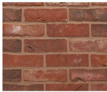
Red facing brickwork
