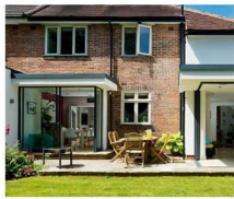
Full height window to rear bedroom
